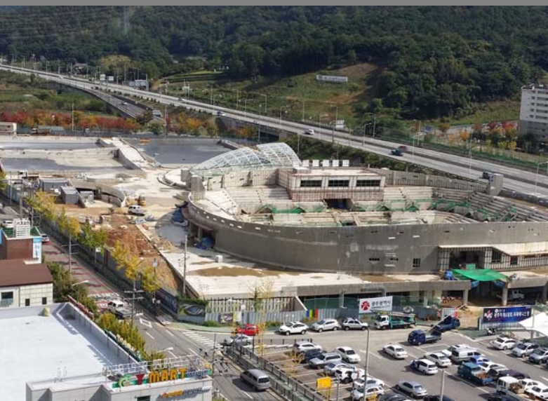
Construction site of Jinwol International Tennis Court (November 2014)
