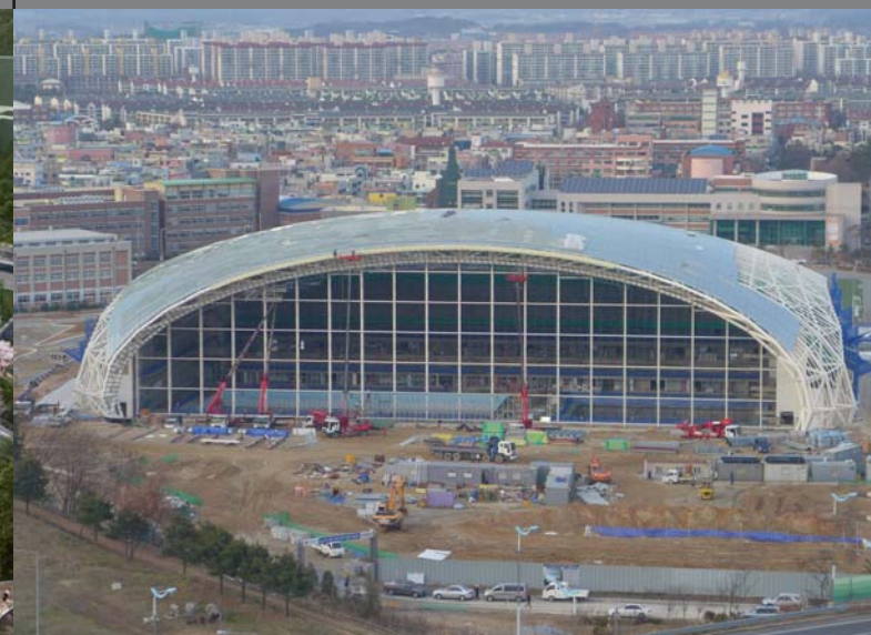
Construction site of Nambu University International Aquatics Center (December 2014)
