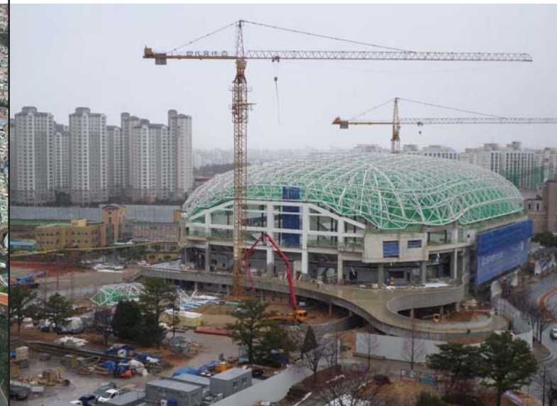
Construction site of Kwangju Women's University Universiade Gymnasium (November 2014)
